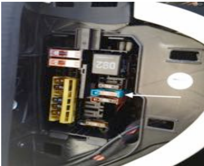
Fuse plugged in on a 2015 C class
