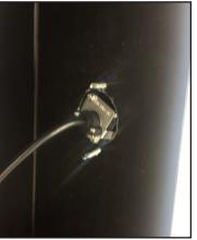
5.3- Slide harness and camera through hole, then fix in place with 2 Tek screws.
